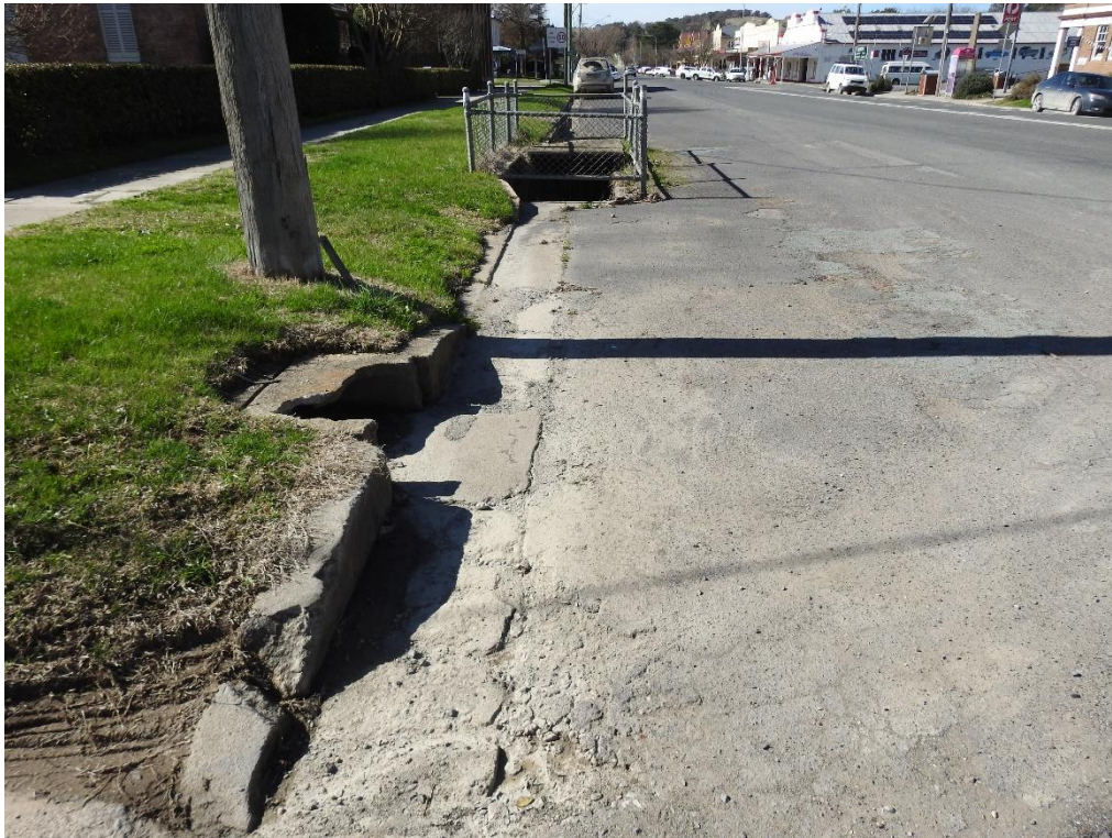
Figure 2. Image from Yass Street showing the location of the discharge point in front of the power pole from the existing easement that traverses between Yass Street and Biala Street, and the fenced stormwater pit compound in front of 105 Yass Street where the proposed inter-allotment stormwater drainage system will discharge.
